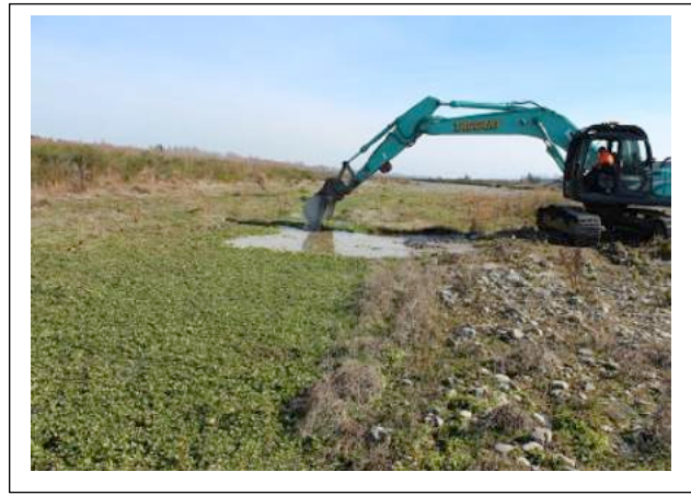
Clearing herbaceous weeds from Groyne 1 seepage site
