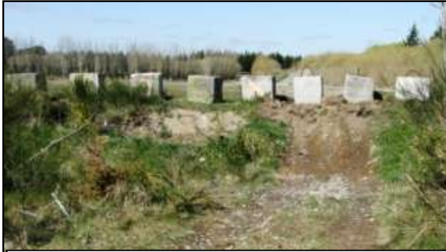
Concrete blocks preventing vehicle access to riverbed.
